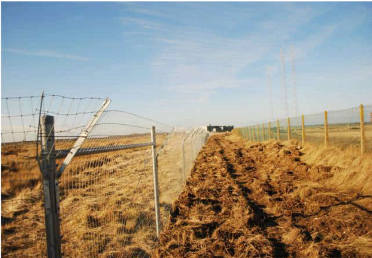
Figure 6-1: A photograph of the completed LBBG compensation measure fence installation
